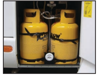
Installation using a bracket in the cylinder compartment should use a 0.6 metre hose
